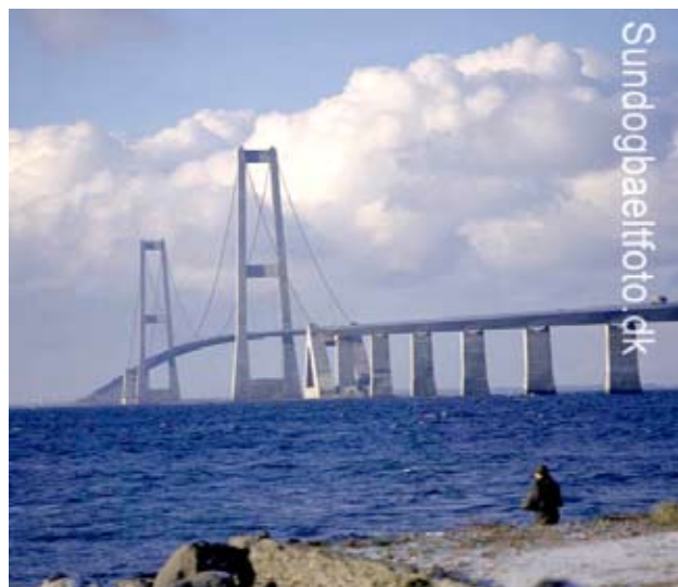
Taller and three times longer than San Francisco's Golden Gate Bridge, Denmark's Great Belt Bridge is a landmark engineering achievement and a vital link for people traversing Denmark.
